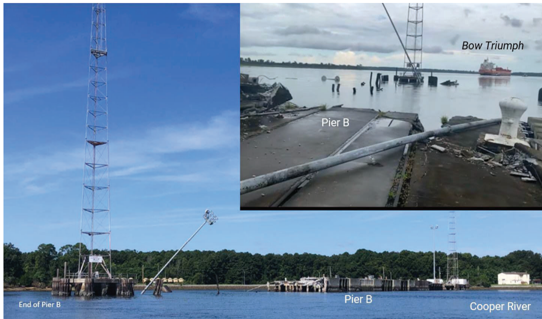
Figure 6 Joint Base Charleston Pier Bravo damage facing west. Inset: Witness photograph taken shortly after the contact facing east. (Photo: USACE, Inset: Jacob Wall)
